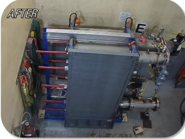
Carbon steel frame secured to heat exchanger skid plates.
