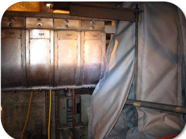
Pressurizer surge line located in a tight spot between the steam generator, the wall, and other interferences.
