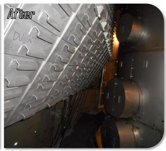
Fully modular—all supports, frames, and lead panels loaded by hand.
