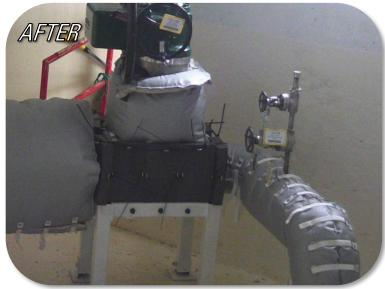
2" (25 mm) thick magnetic shield tiles for valve. Integrated hardware allow tiles to be tied together. 640 lb (290 kg) total shielding package supported by steel frame and secured with cable ties.
