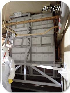
Significant amount of shielding required in incore rooms for Units 1 & 2. The shielding needed to effectively block entire room.
