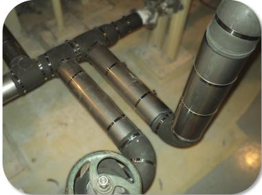
Solid Lead jacketed in stainless steel were used for the straight sections.
